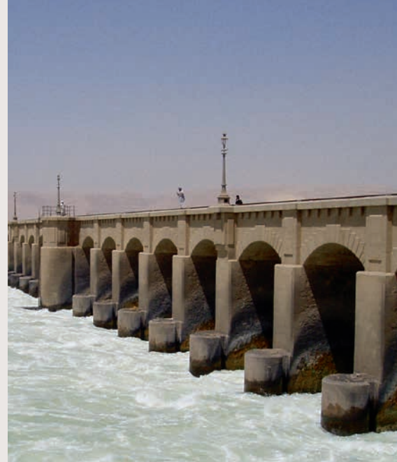
New Naga Hammadi Dam
